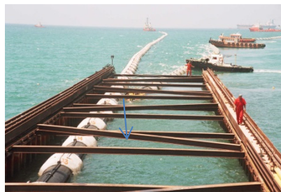
Intake Pipes Laying, Ashkelon
