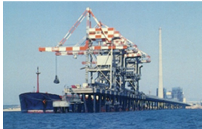
Hadera Coal Unloading Pier
