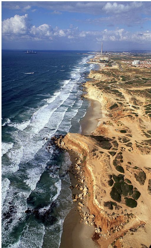
Figure 4. Beach and cliff erosion at Havazelet Hasharon coastal sector north of Netanya
