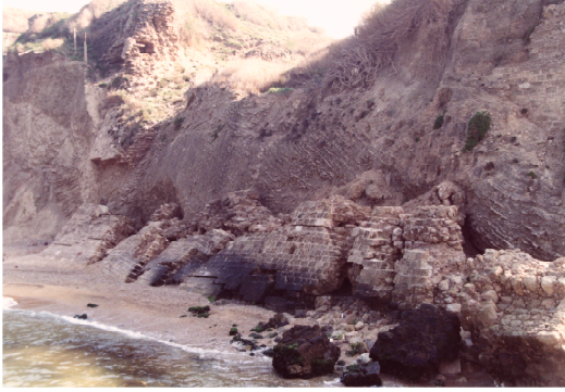
Figure 2. Collapse of the Apolonia fortress wall at Herzliya due to severe beach and cliff erosion
