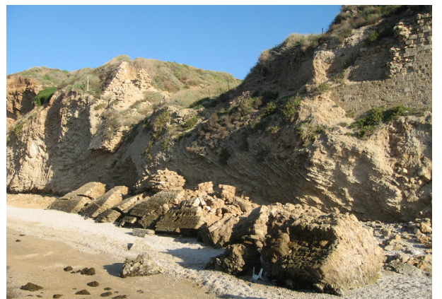
Figure 8. Collapse of Apolonia fortress wall due to severe beach and cliff erosion
