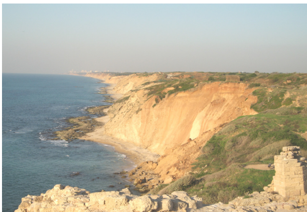
Figure 7. Severe coastal and cliff erosion north of Apolonia ancient fortress, at Herzliya
