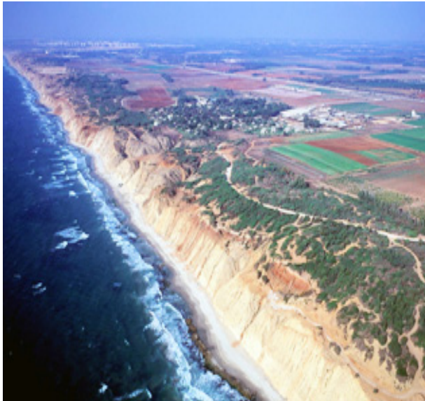
Figure 9. Beach and cliff erosion at Shefaim-Gaash coast endangers residents on cliff top.
