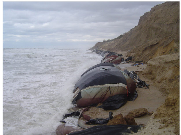
Figure 6. Failure of the geotextile tubes protection, probably due to their impermeable rubber cover.
