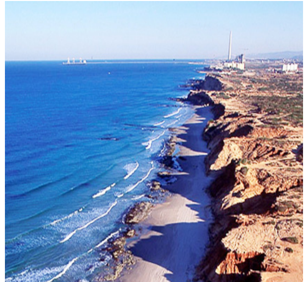
Figure 10. Coastal and cliff erosion at HaSharon sector, north of Netanya.
